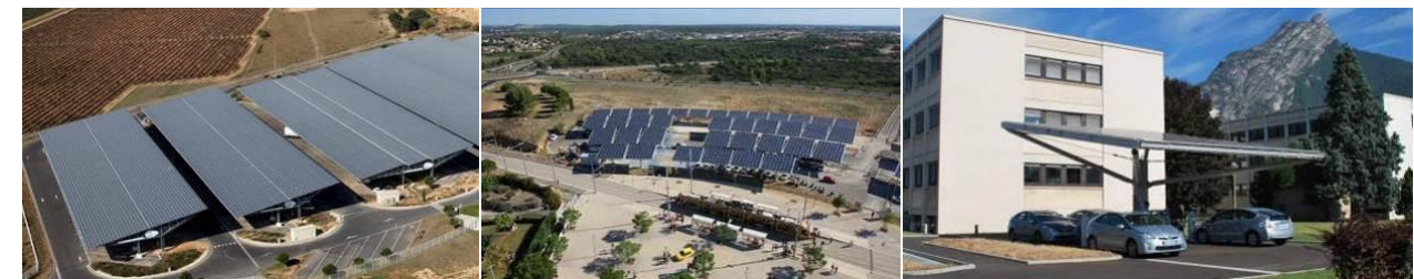
Figure 9 : Illustration des ombrières photovoltaïques (source : QUADRAN, 2015)
